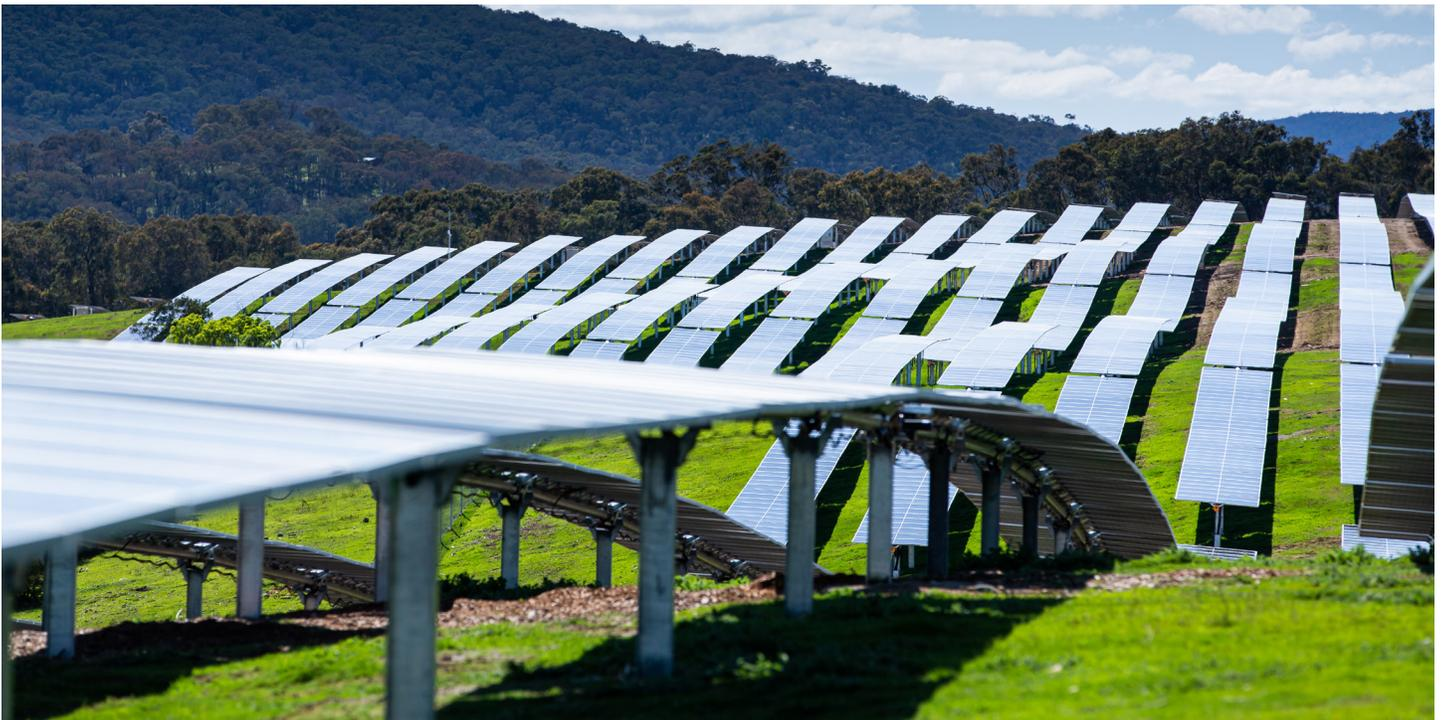
NX Horizon-XTR, the field-proven solar tracker for hilly terrain with more than 5 GW deployed on multiple continents
