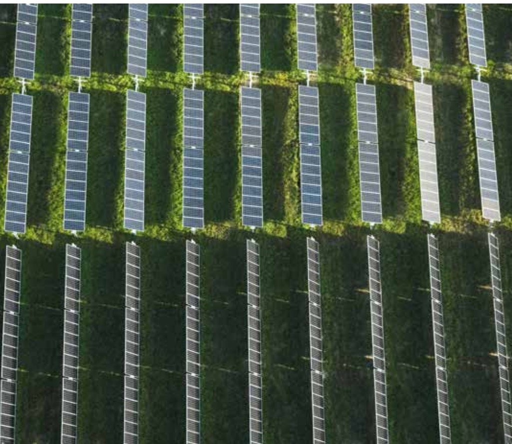
SHADE AVOID IN ACTION In this aerial photograph, TrueCapture's Shade Avoid mode is turned on for the tracker rows with unshaded modules (on top) and turned off for those trackers experiencing row-to-row shading (on bottom).
